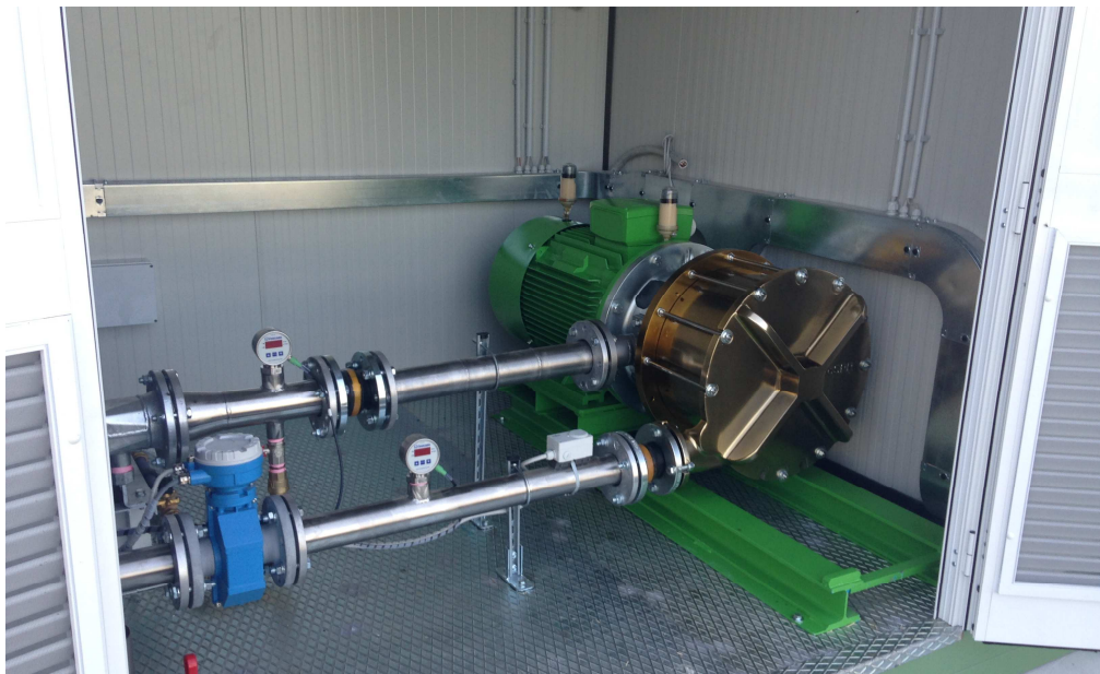
Picture of installed BipSPR unit in Italy
