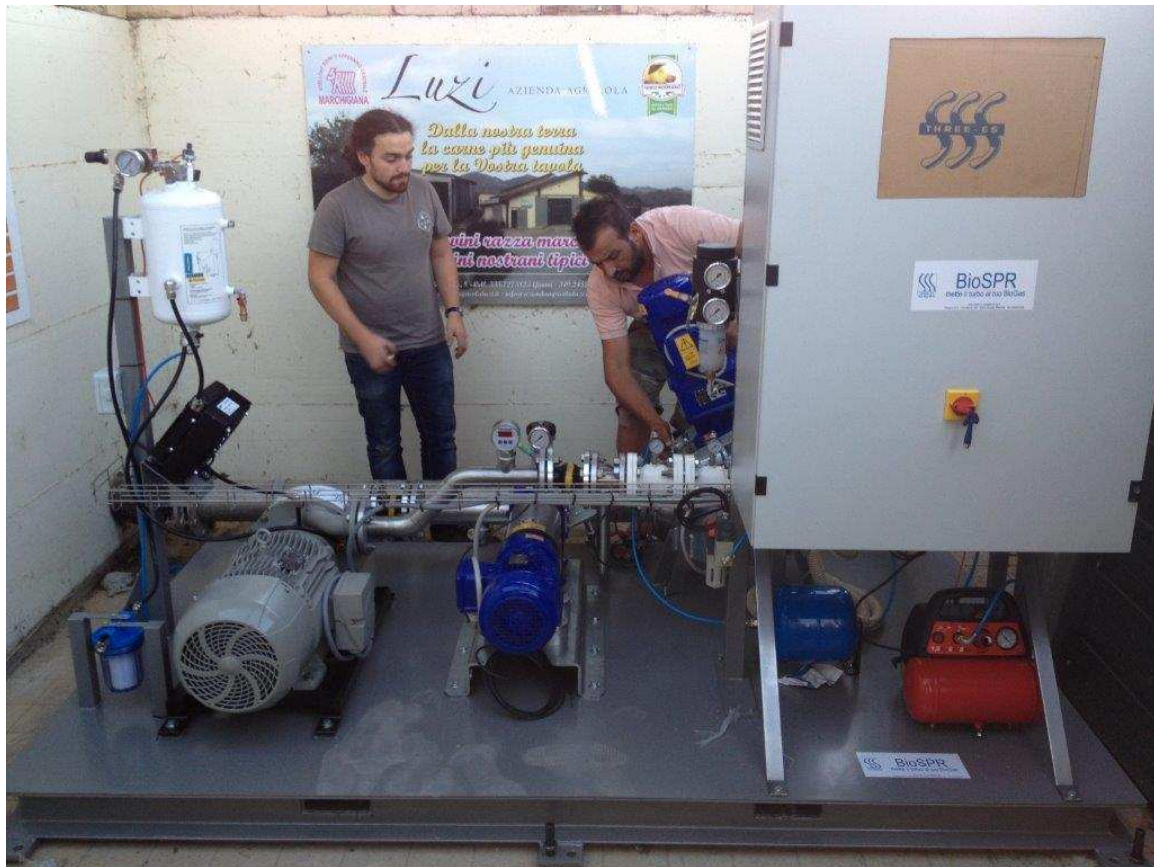
Picture of Biogas Unit Skidded for Installation
